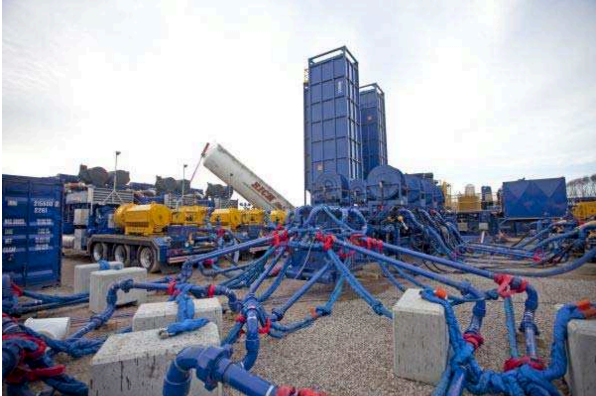
Picture 2: Source Cuadrilla Resources - Image of Preese Hall.
